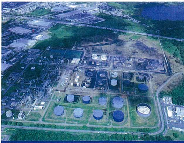
Figure 2. Aerial view of the Caribbean Petroleum facility after the explosion.
